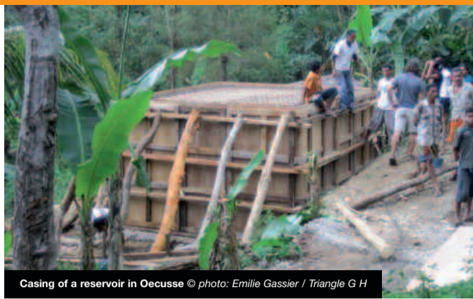
Casing of a reservoir in Oecusse © photo: Emilie Gassier / Triangle G H
