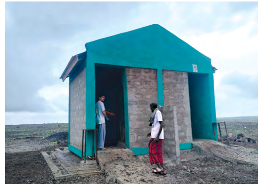
Assessment of communal sanitation infrastructure in an informal internally displaced persons (IDP) settlement in Mahi Rasu, 2025. © TGH
