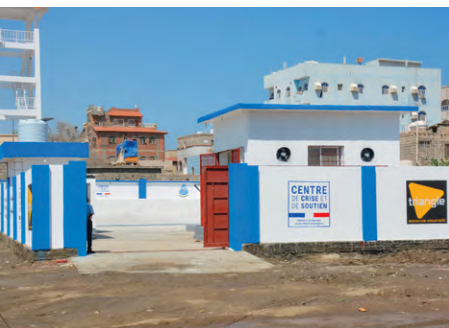
Wastewater treatment plant at Al-Gamhouriah Hospital, rehabilitated by TGH, 2025. © TGH
